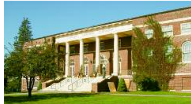
Existing Sargent Gym
