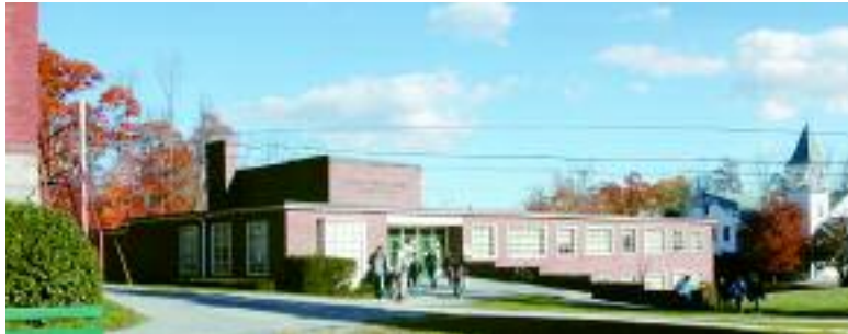
Treat Science Center, Existing Building
